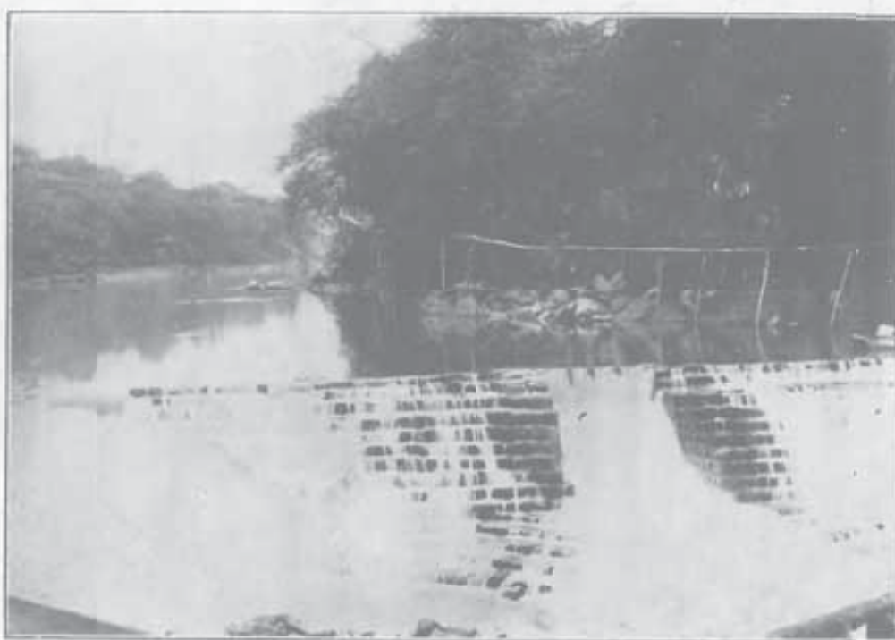
Method of damming small Streams to ensure sufficient water for Boat Traffic down to the main R - Bamboo lead pipes may be seen on the right.
