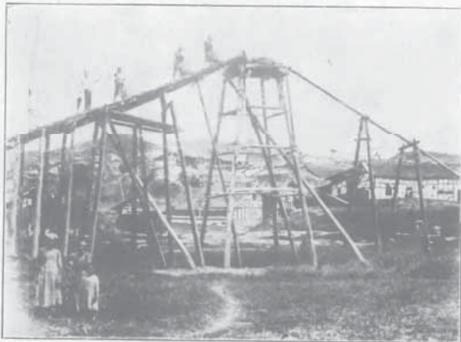
Codies Carrying Brine up the Trestle Work to the Nests into which it is Poured and allowed to Run to the Boiling Pans. The Bamboo Pipe-line leads off to the right.
