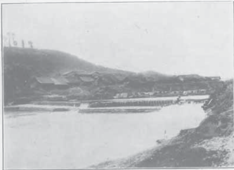
Often Temporary Dams are made by Filling Salt Bags with Sand. The Runway for the Boats is to the Right. During High Water the Dam is Washed Away.
