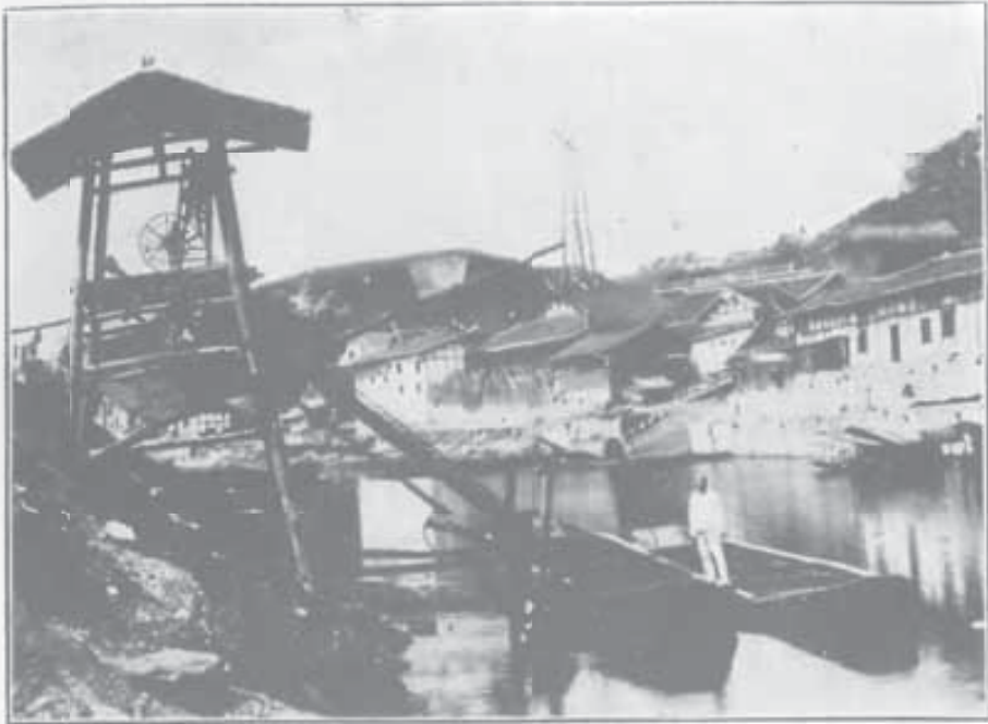
Arriving at the Boiling Pans, Treadmills are used to Draw the Brine, by Man Power, up to the Pans. A man can be seen working a treadmill and drawing the brine up to the level of pans.
